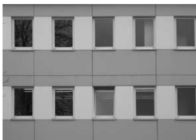
Obstoječa stavba pred prenov
